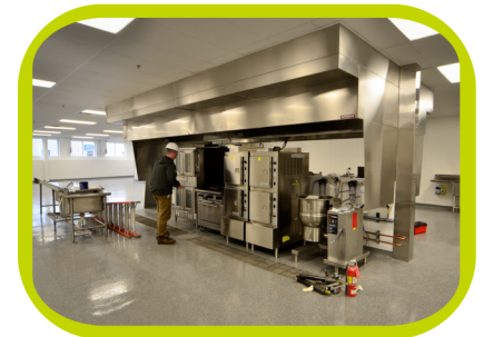
The new kitchen being constructed at Wilson Ave!
